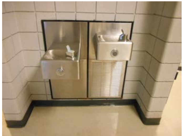
ADA Compliant Electric Water Cooler -1990 Original Construction
