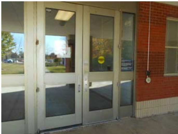
ADA Compliant Power Assisted Door-1990 Original Construction
