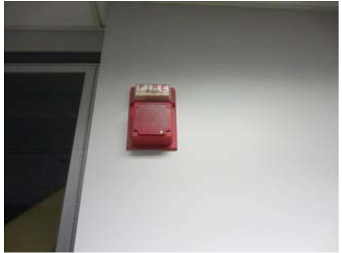
Fire Alarm System Audible Horn and Strobe Indicating Device
