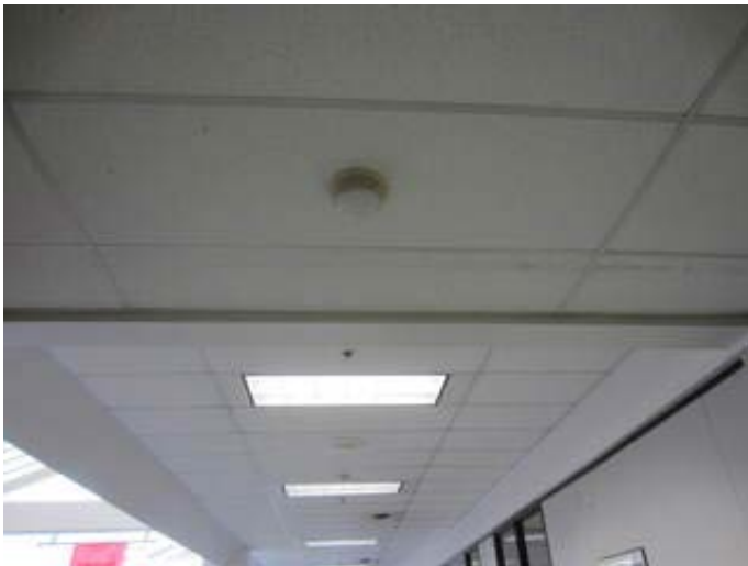
Security System Motion Sensor
