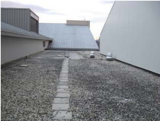
Ballasted Roof
