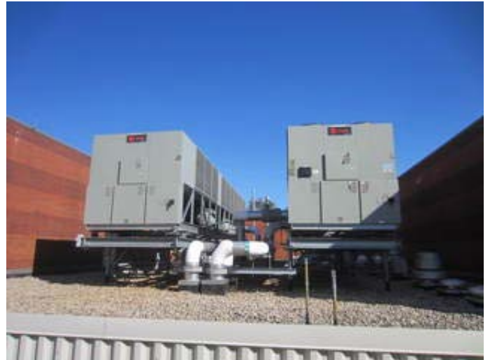
Air Cooled Helical-Rotary Liquid Chillers
