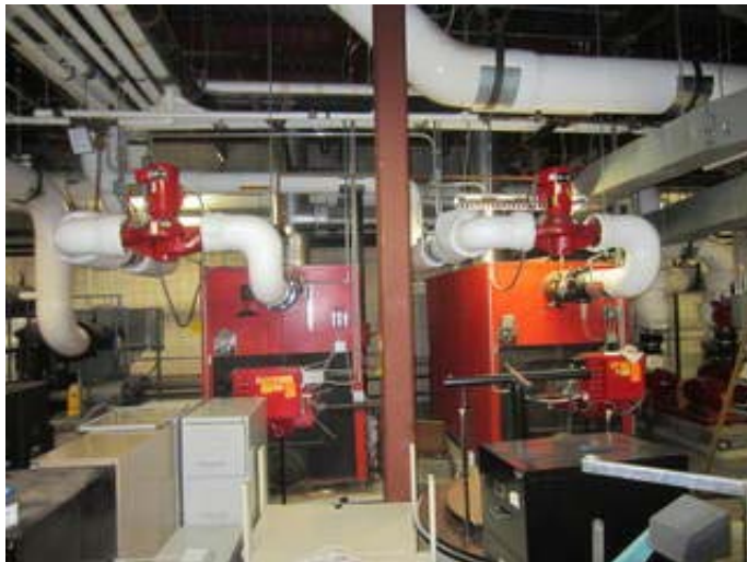
Natural Gas Fired Heated Water Boilers
