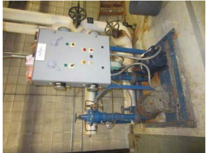
Incoming Domestic Water Service Line Booster Pump
