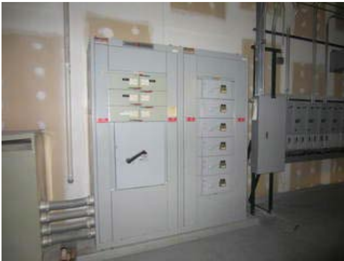
Main Electrical Distribution Panel
