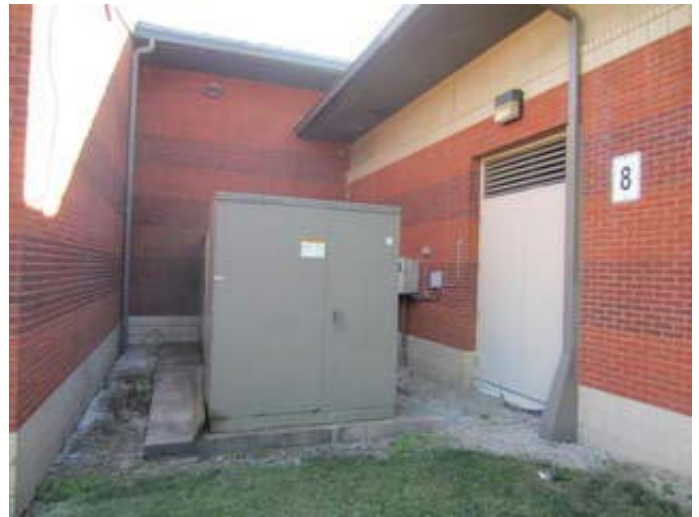
Pad Mounted Transformer
