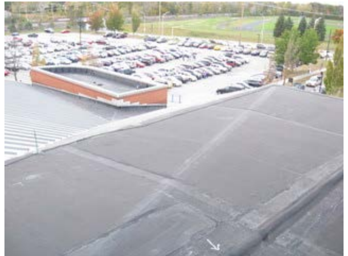
Standing Seam and Membrane Roofing
