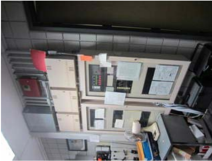
Fire Alarm System Control Panel
