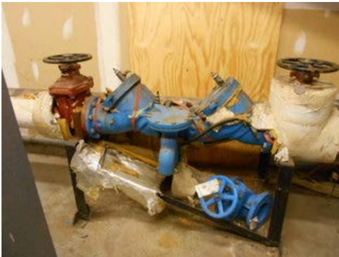
Reduced Pressure Backflow Preventer
