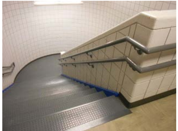
Compliant Enclosed Egress Stairway
