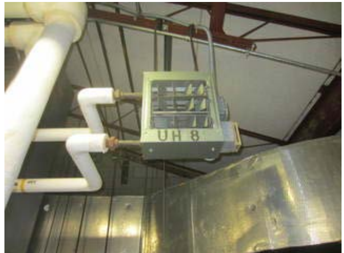
Heating Water Unit Heater
