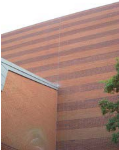
Brick Veneer and Control Joint
